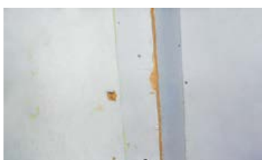
Figure 24 Chrysotile paper on fibreboard boxing
