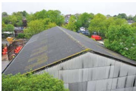
Figure 32 Asbestos cement roof and cladding
