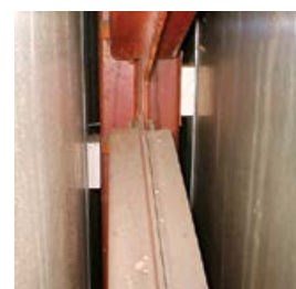
Figure 22 AIB offcuts used as packers around column in CLASP building
