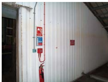
Figure 38 Chrysotile/bitumen coating under metal cladding
