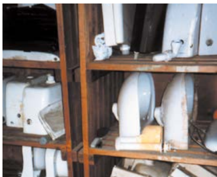
Figure 40 Asbestos-reinforced toilet cistern
