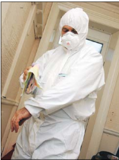
Cleaning with damp rag using patting action
