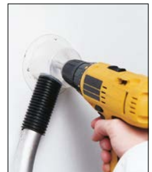
Control measures: shadow vacuuming and using a drill cowl as local extraction
