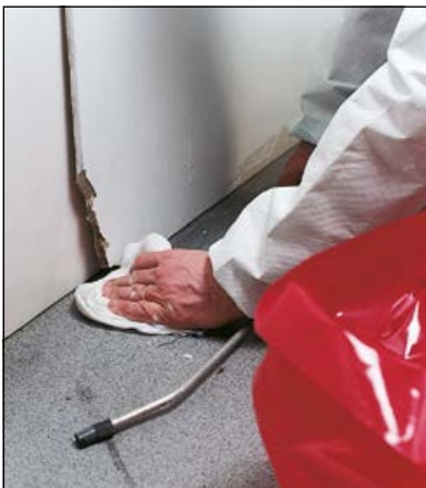
Wiping up debris with a damp rag
