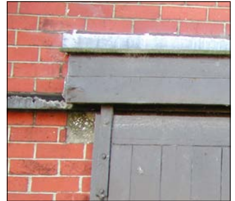
Built-up bituminous roofing and bituminous asbestos fabric over a doorway
