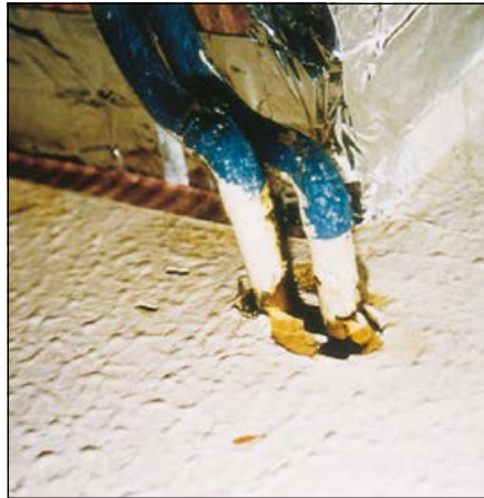
External AC panels
