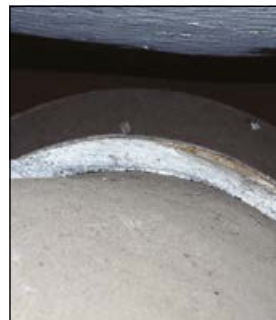
Joint packing on a flue
