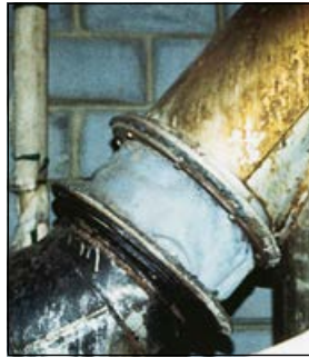
Connectors may be clipped or riveted
