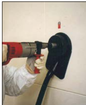
Control measures: shadow vacuuming and using drill cowls as local extraction
