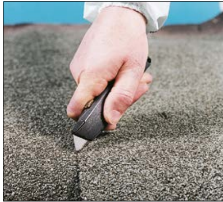
Cut and remove manageable sections
