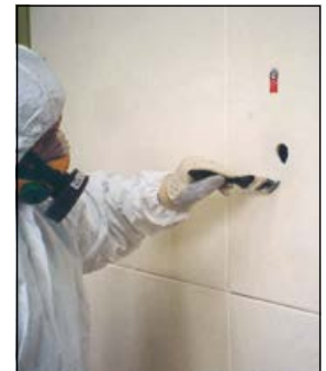
Seal the drilled edge with sealant
