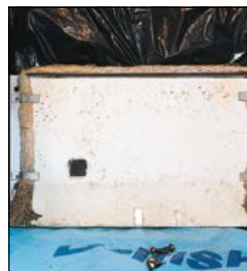
Some examples of rope seals found on boilers
