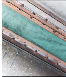
Connectors may be clipped or riveted
