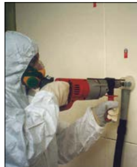
Control measures: shadow vacuuming and using drill cowls as local extraction
